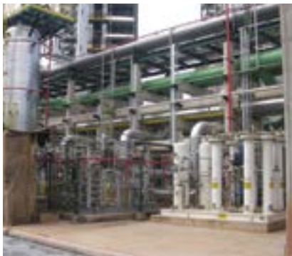
XEBEC 3100 IN BRAZIL Ethylene cracker off-gas hydrogen re-used in polyethylene production
